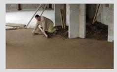
Developed over many years Supaflo\* is at the forefront of screed technology. A flowing screed flooring solution based on a calcium sulfate binder, it provides significant additional benefits such as speed of application, excellent surface finish, accuracy of placement and finishing, reduced thickness and a substantial reduction in movement joints.
